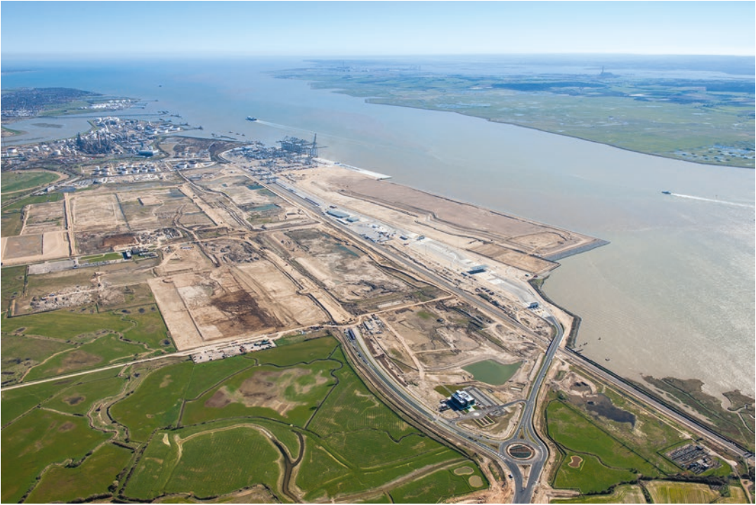
Fig. 26.1 Construction work in progress at the London Gateway Port development on the Essex coast in the Thames Estuary, giving an impression of the area affected and the potential impact on the historic environment. © Historic England Archive, Damian Grady
