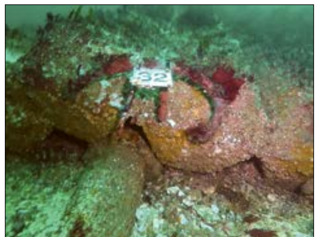
Figure 6.2. Pictures of iron shells and concrete mattresses used to protect an unburied cable at the Paimpol-Bréhat tidal turbine test site in France. The picture on the left was taken one month after the installation of the concrete mattress in 2013 (photo courtesy of Olivier Dugonay, Ifremer), and the picture on the right was taken six years later during a video survey (photo courtesy of Ifremer).
