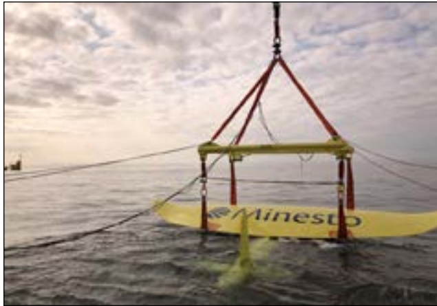
Figure 3.4. Minesto's Deep Green 0.5 MW tidal kite being deployed at Holyhead Deep, in Anglesey, Wales. (Photo courtesy of Minesto)
