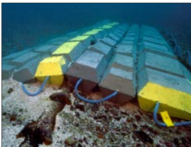
Figure 6.2. Pictures of iron shells and concrete mattresses used to protect an unburied cable at the Paimpol-Bréhat tidal turbine test site in France. The picture on the left was taken one month after the installation of the concrete mattress in 2013 (photo courtesy of Olivier Dugonay, Ifremer), and the picture on the right was taken six years later during a video survey (photo courtesy of Ifremer).
