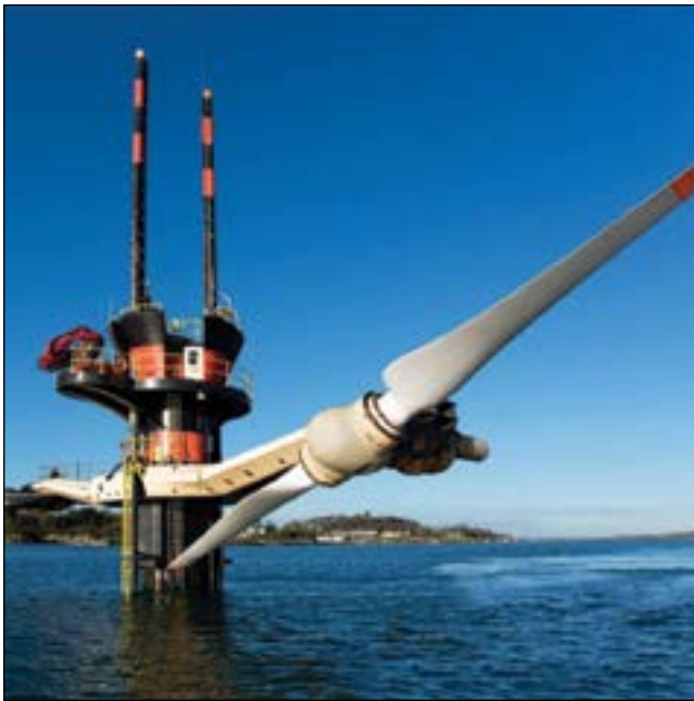
Figure 3.3. The SeaGen tidal turbine when installed in Strangford Lough, Northern Ireland. (Photo courtesy of SIMEC Atlantis Energy)
