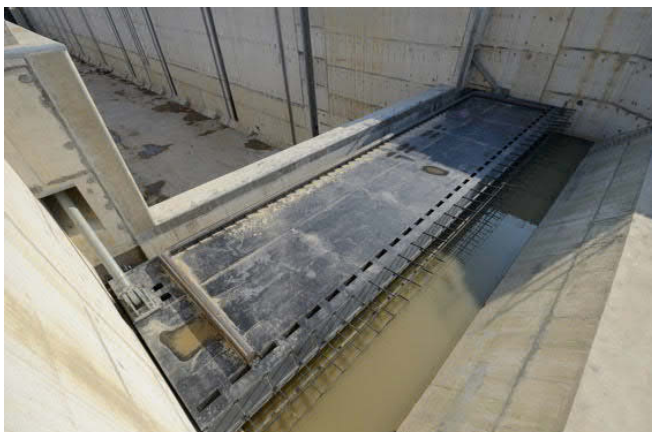
Fig.5: Upstream flap gate – © Greisch
