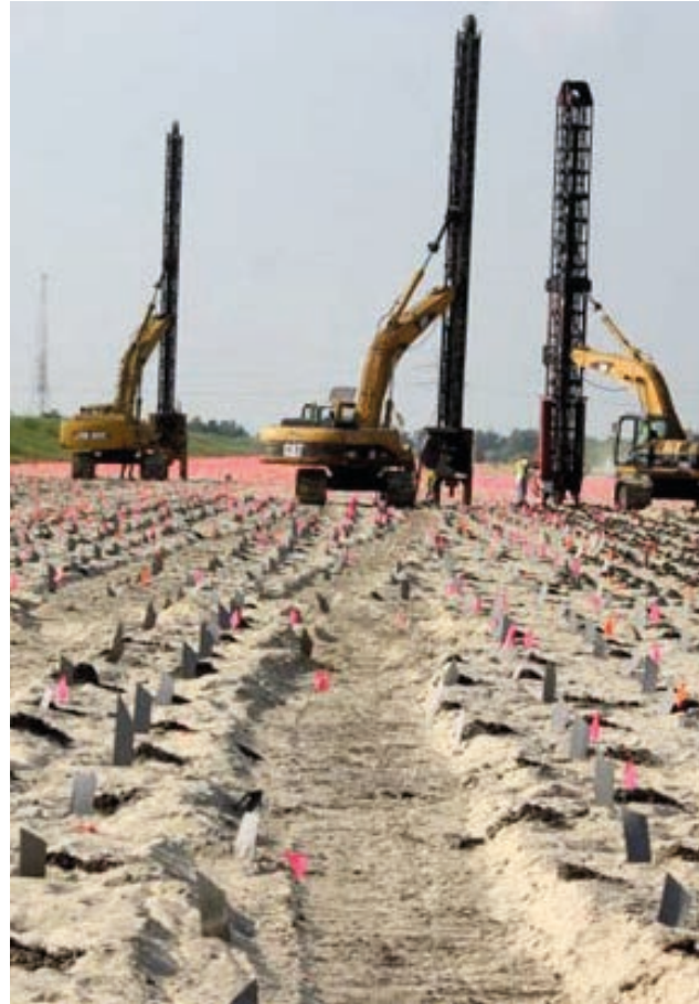
Figure: Wick drains are installed using specialized equipment called stitchers.
