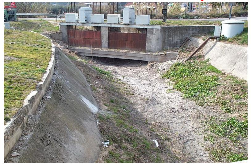
• Inlet structure to compartments in the flood plain
