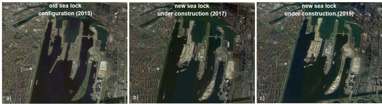
Fig. 4. Comparison among the (a) old configuration of sea lock (2015), (b) new configuration of the sea lock at the beginning of the construction (2017), (c) a recent status of the sea lock construction (2019). Photos credit to Google Earth.
