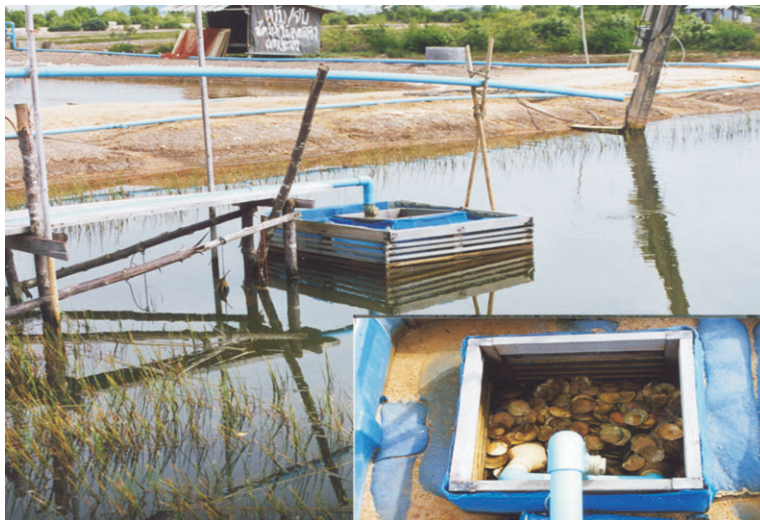
Fig. 29. Treatment pond for small scale water recycle pond using integrated physical and biological technology.
