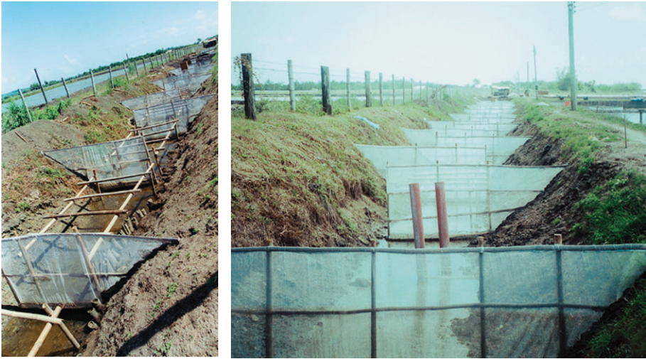
Fig. 5. Baffles in the settling pond.
