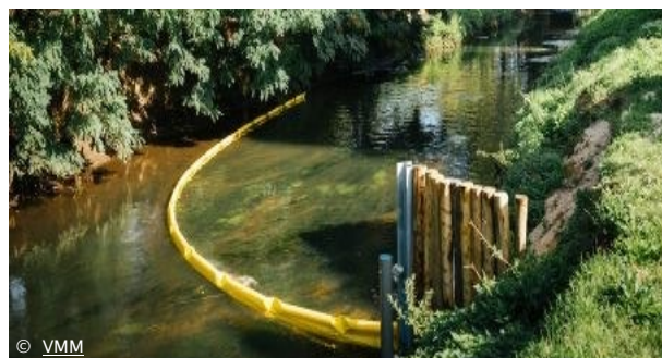
Figure 23 : One of the plastic catchers installed by VMM as part of the LIVES project
