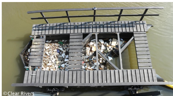
Figure 22 : The litter trap, a Clear River's initiative, installed in the port of Brussels
