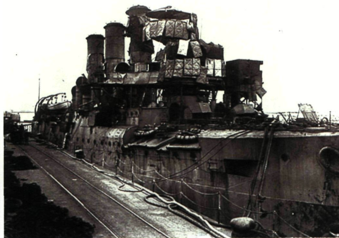
H.M.S. Vindictive, at Dover, -from Zeebrugge.
