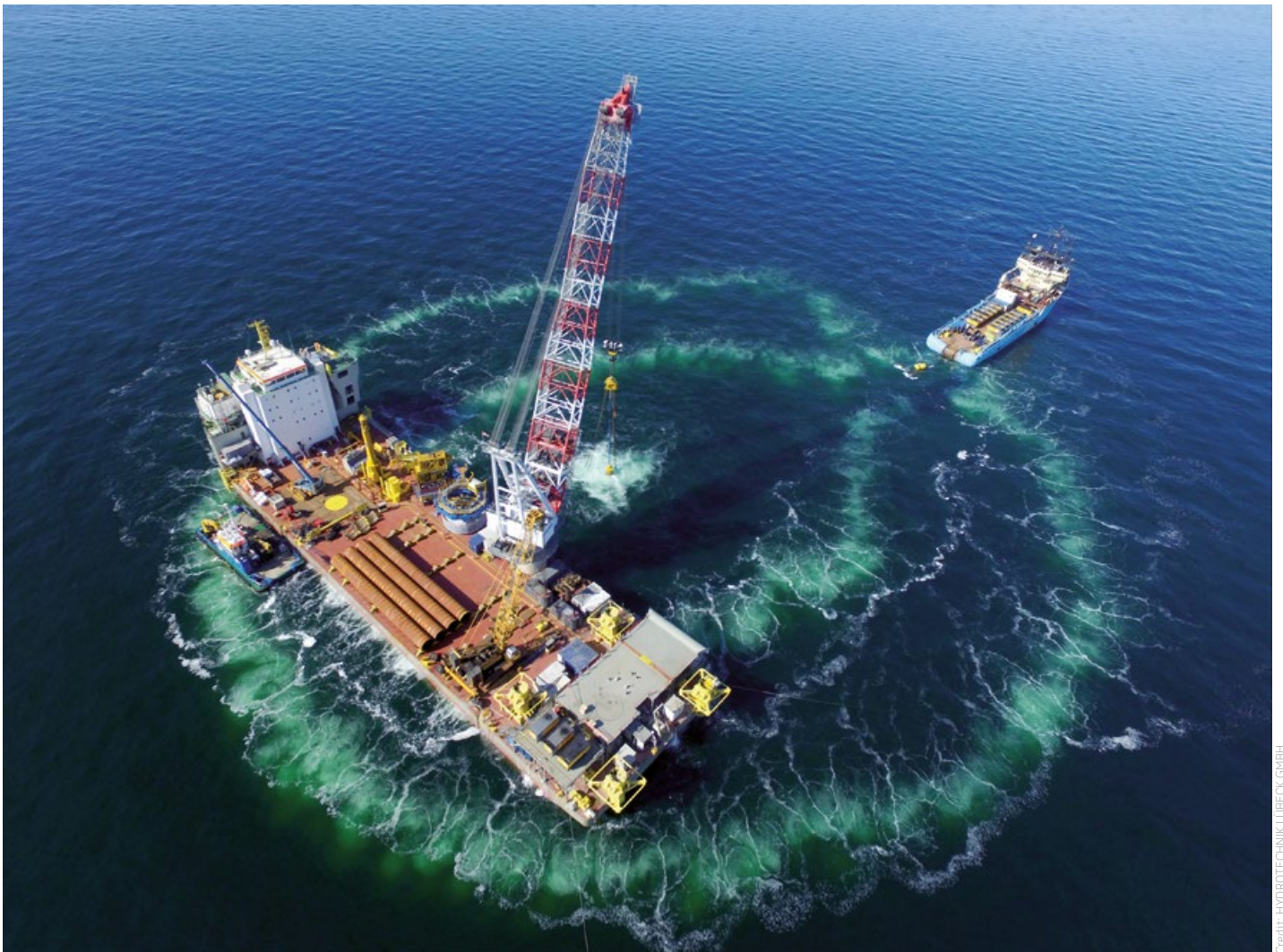
Double Big Bubble Curtain in action, used to mitigation sound propagation from pile-driving.
