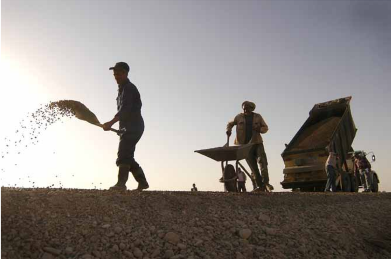
Workers on a road construction site
