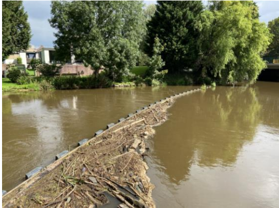
Figure 7: Litter trap in the Roer in Roermond (source: https://litterfreeriversandstreams.eu/litter-traps-in-roer-en-geul/ )
