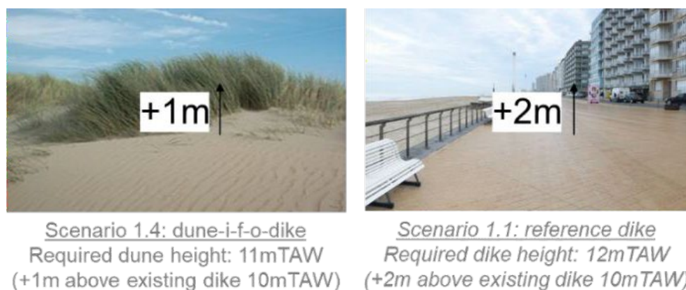
Figure 1: Estimated height required to protect the coast in the future against a sea level rise of +1.5m: for a dune-in-front-of-dike (left) and for a reference hard dike (right).
