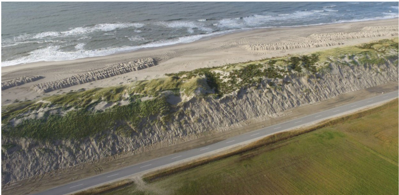
Figure 2: Removed sand for the road and back dune and placed in different patterns on the beach.
