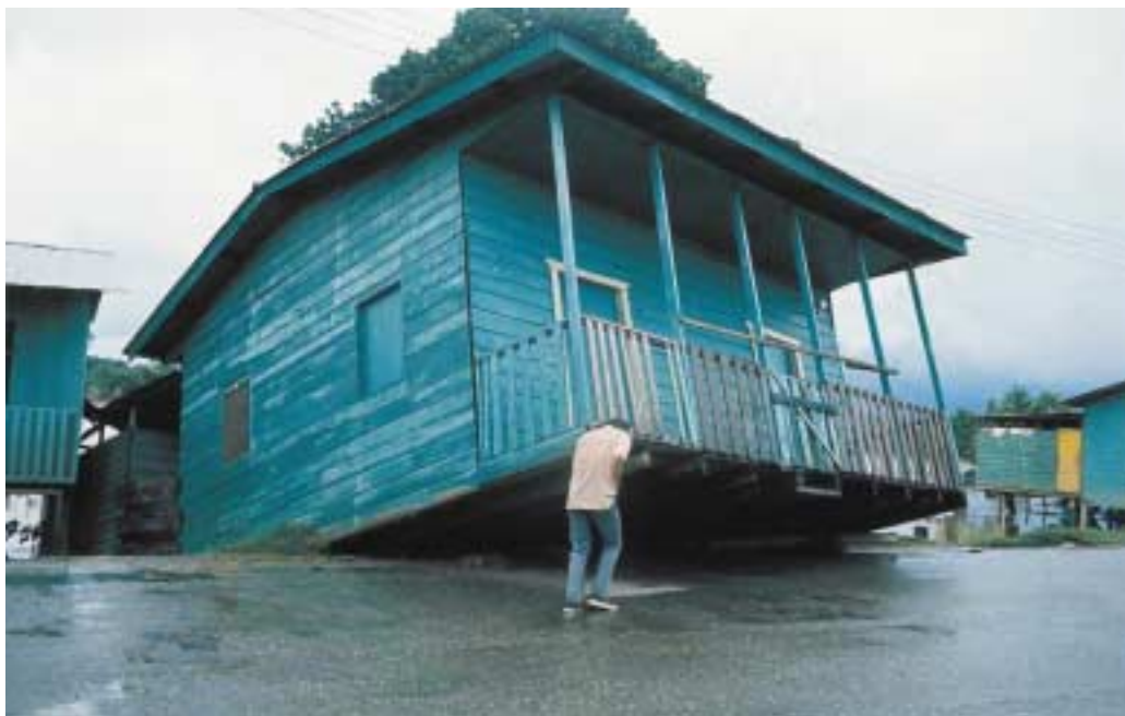
(a) above: a house uprooted and displaced. (b) below: two buses bogged down on a road flooded by heavy rains.
