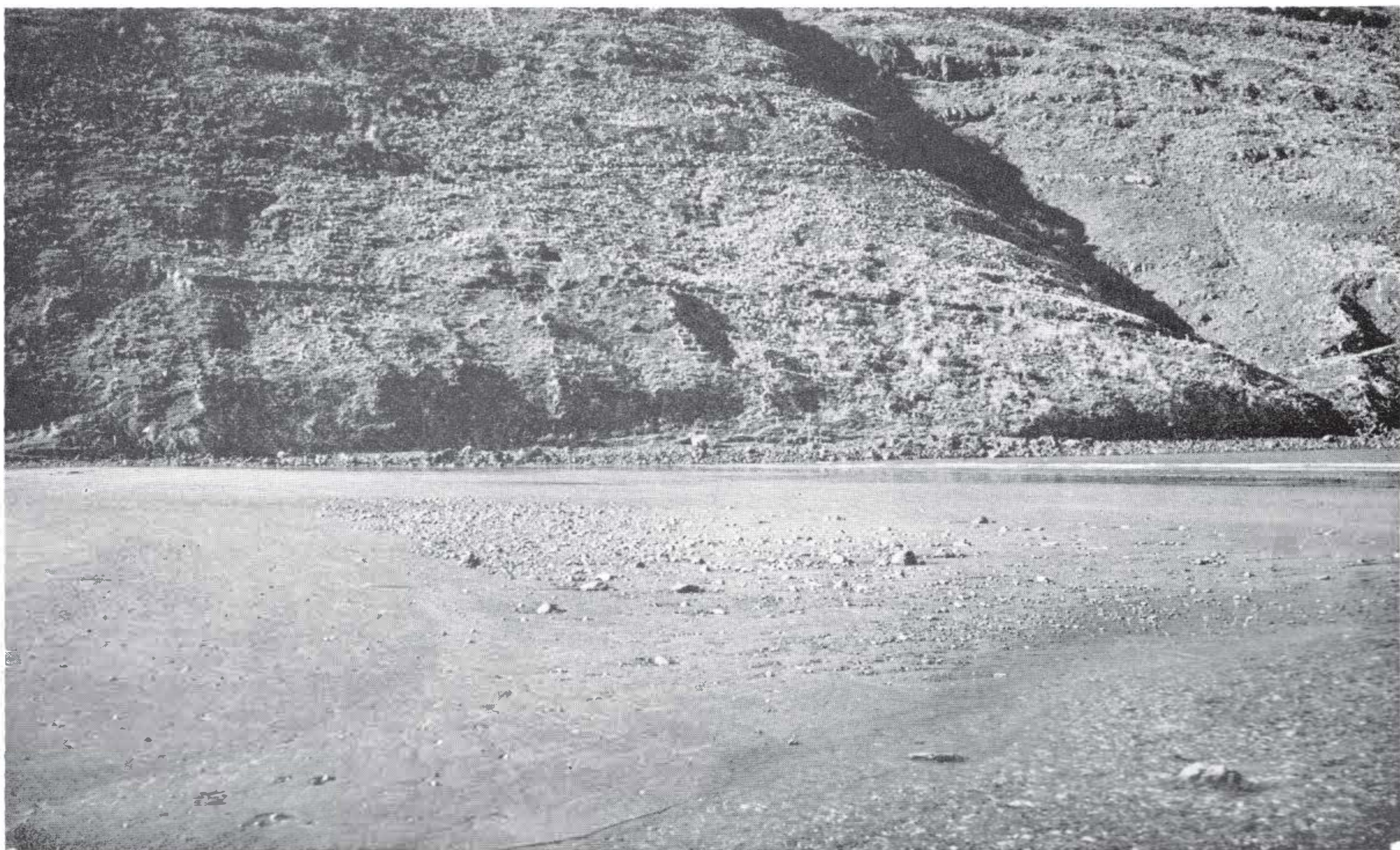
Figure 21 Beach foundation exposed by winter wave action at Peraki Bay.
