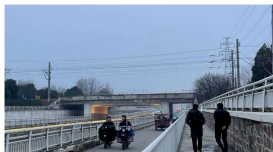
Figure 5. An underpass in Kaifeng
