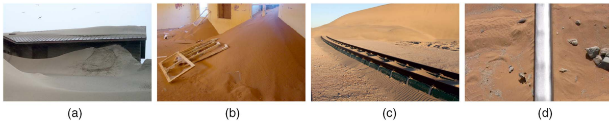
Fig. 1. Windblown sand effects on structures and infrastructures: (a) buried houses in Waldport, Oregon; (b) in In-Salah, Algeria; (c) buried railway track in Namibia; and (d) rail deformation. [Reprinted (a–c) from Engineering Structures , Vol. 178, L. Raffaele and L. Bruno, “Windblown sand action on civil structures: Definition and probabilistic modelling,” pp. 88–101, © 2019, with permission from Elsevier; reprinted (d) from Journal of Wind Engineering and Industrial Aerodynamics , Vol. 177, L. Bruno, M. Horvat, and L. Raffaele, “Windblown sand along railway infrastructures: A review of challenges and mitigation measures,” pp. 340–365, © 2018, with permission from Elsevier.]
