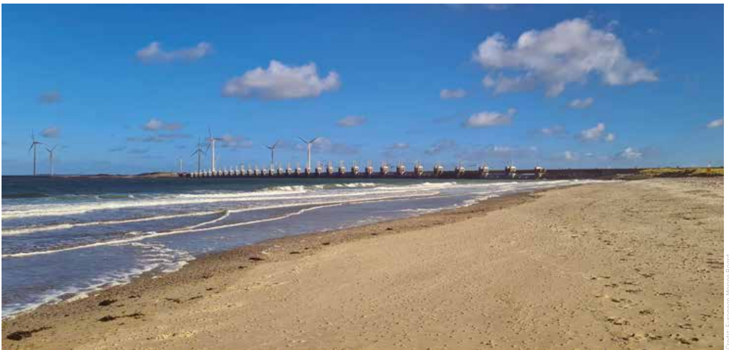
Figure 3.3 Oosterschelde tidal range power plant in the Netherlands.
