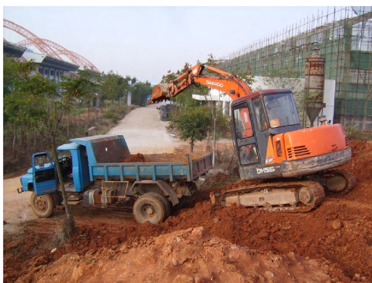
Figure 20 Excavator and Truck in the delivery
