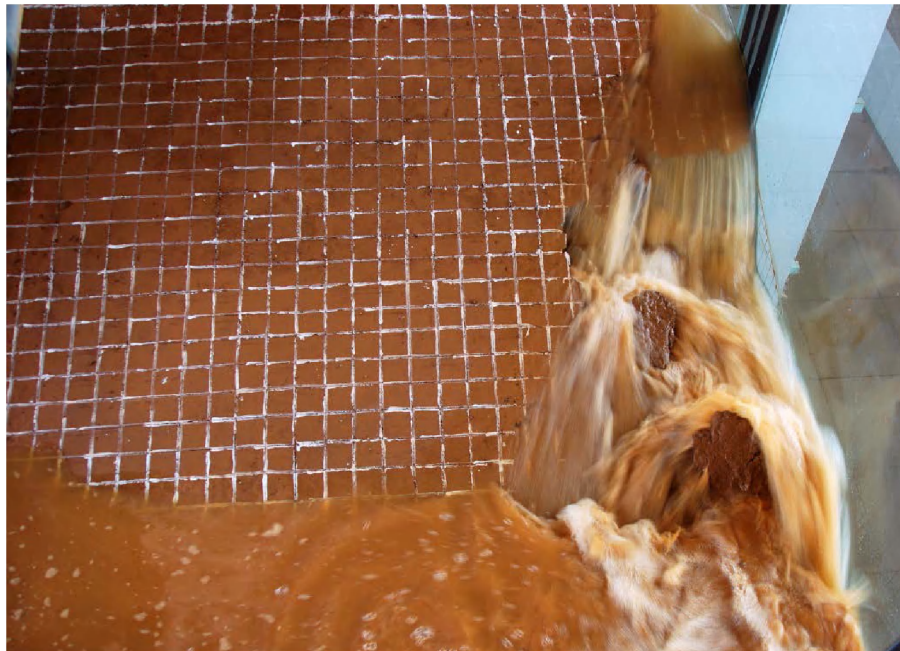
Figure 39 Photo of Headcut Erosion
