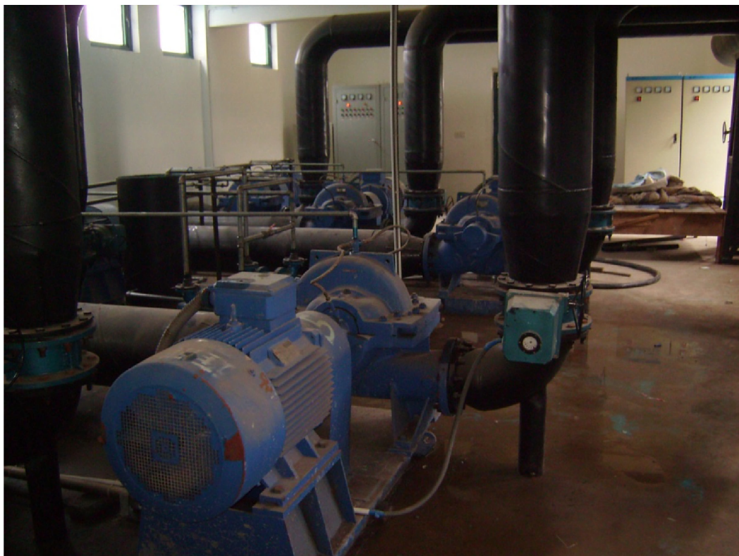
Figure 7 Flume Pumps Layout
