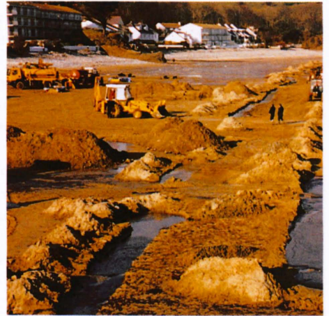
Trenches at Saundersfoot, 28 February 1996 (E Bent)
