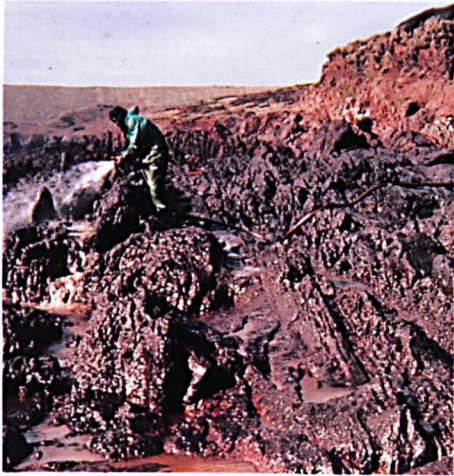
High-volume water flushing to displace oil on rocky shoreline, between Wiseman's Bridge and Amroth (ITOPF)
