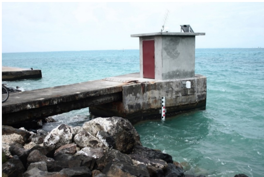
FIGURE 2 The typical tide gauge geodetic station of Tubuai (austral archipelago, see Figure 1 for location). One can see the RADAR altimeter (vertical corner), the GOES UHF Yagi antenna on the roof as well as the GPS radome and a solar panel.
