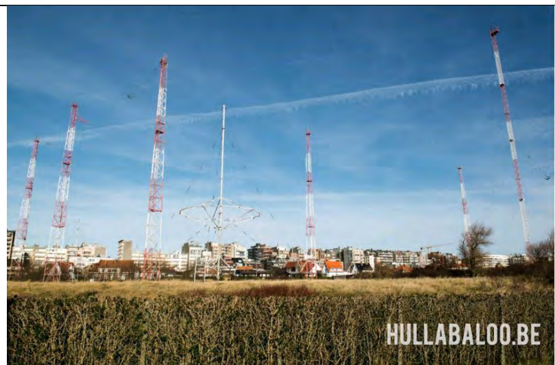
Zendstation "Radio Oostende" © Hullabaloo
