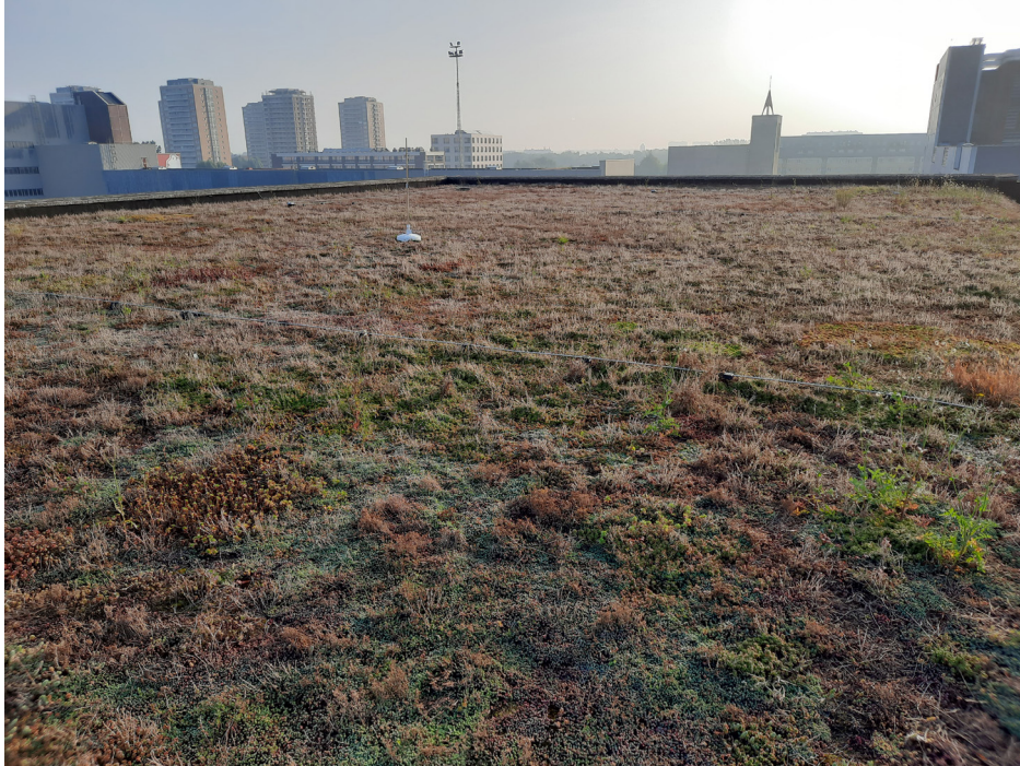
Fig. 1. Green roof BRA (Brandweer, Antwerpen), Antwerp, Belgium. © Jeffrey Jacobs.
