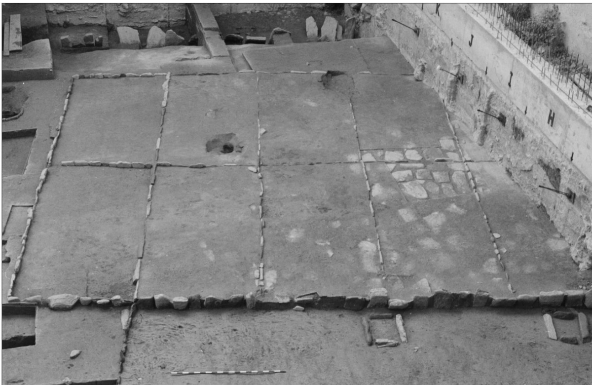
Figure 34 Well-preserved crystallization ponds in the west sector of the O Areal salina (Vigo, Spain). In total 8 complete 5 x 2.5m compartments with a carefully constructed stone and clay pavement delineated by ca. 10cm high stone slabs can be observed (Castro Carrera, 2006, fig. 11)
