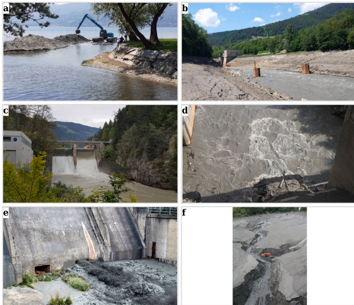
Fig. 1. Examples of sediment removal by: a) Mechanical dredging (Lago Maggiore, Lombardy, Italy); b) emptied reservoir during sediment flushing operations, c) starting of flushing event closing the upper dam's gate and opening the bottom outlets, d) top view of the water surface immediately upstream of the dam (Pictures b, c and d are taken in Alto Adige, North of Italy); e) pressure flushing f) mechanical dredging (Fusino dam in Valgrosina).
