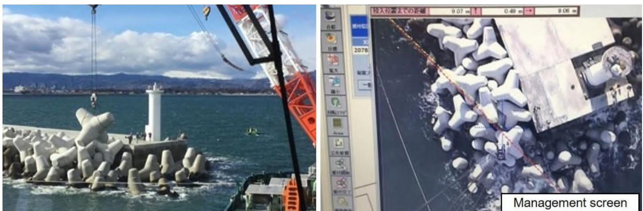
Figure 22: Installation at the target position guided by the management screen
