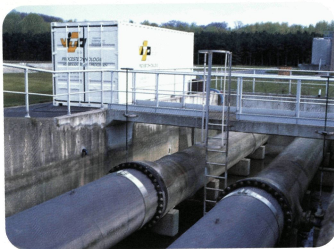
Fig. PRO 2: View of the mobile filtration loop for water applications
