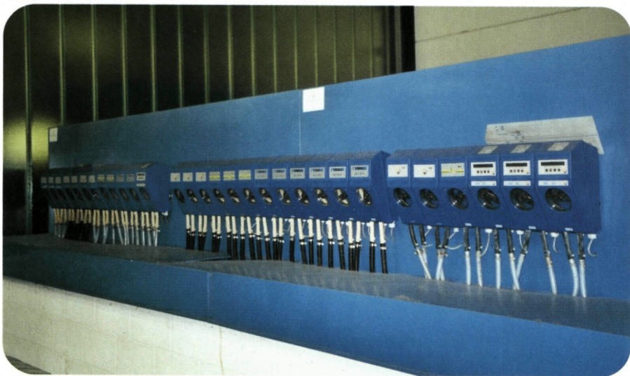
Fig. PPE 2: Example of a 'Best available technique' for the laundry sector: automatic dispensers reduce the detergent consumption and water pollution.
