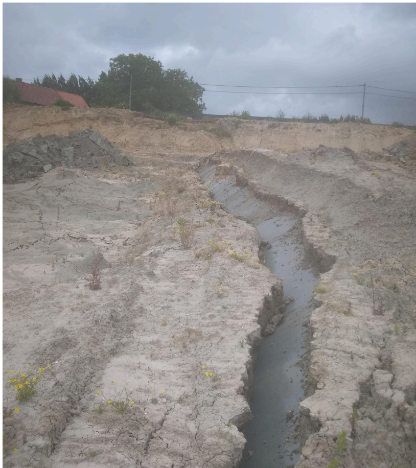
Figure 1. Picture of the fault as observed in the clay pit in Rumbeke (image source: Jan Maertens)
