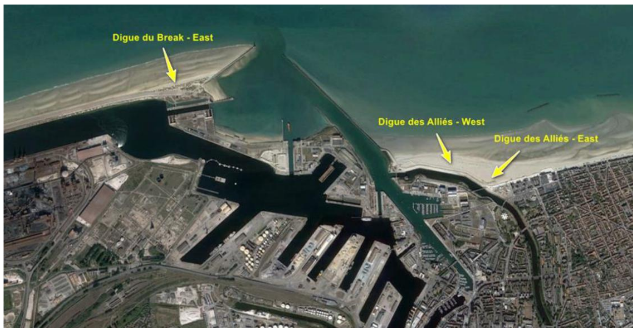
Figure 3: Dunkerque (FR) Demonstrator, at three key locations: Malo les Bains (West and East sections of the Digue des Alliés) and Digue du Break
