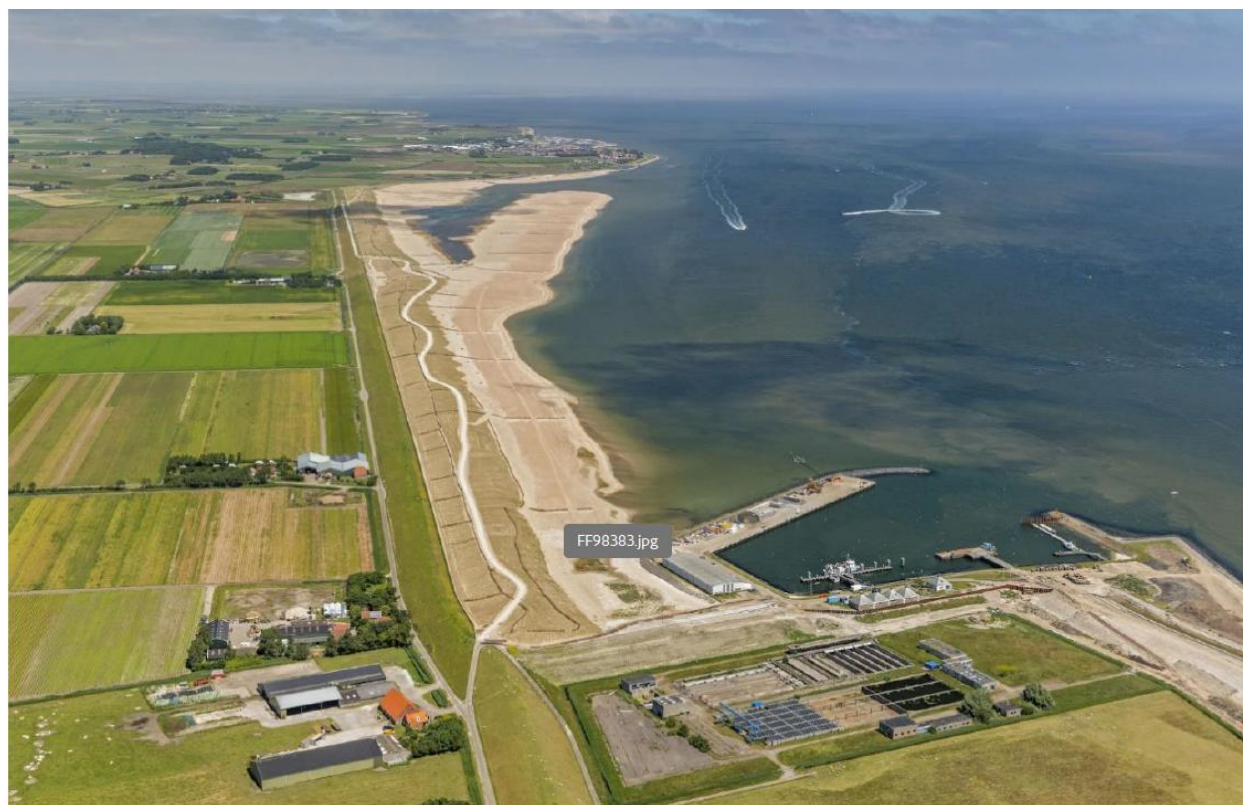
Figure 5: Texel, Prins Hendrik Zanddijk (NL) Demonstrator, Dune-in-front-of-Dike
