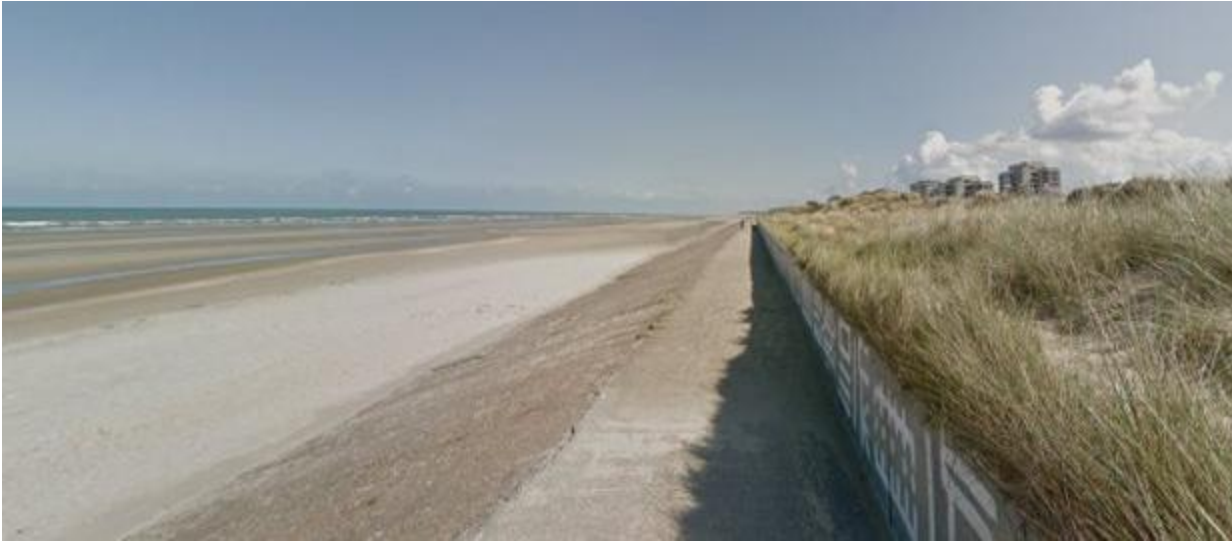
Figure 1-1 Current conditions of the concrete dune reinforcements at the level of Westerpunt (De Panne).
