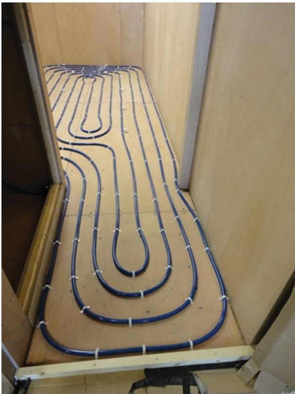
Fig. 7. The floor heating tubes. Photo: JM Services
