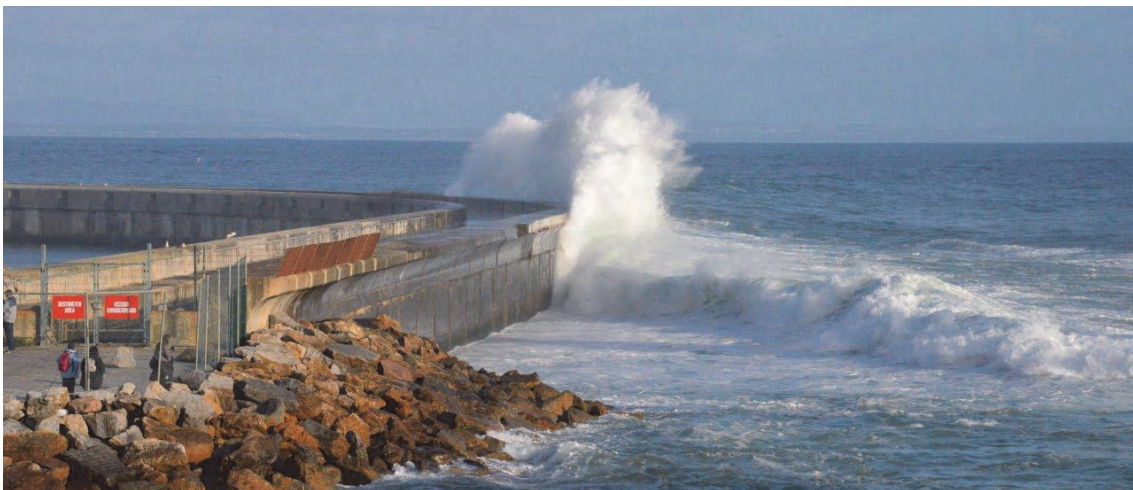
Figure 1.8: Effective fairly significant bullnose at Cascais, Portugal. Waves are breaking on the foreshore and give impulsive wave conditions. There was no wind. Courtesy L. Franco
