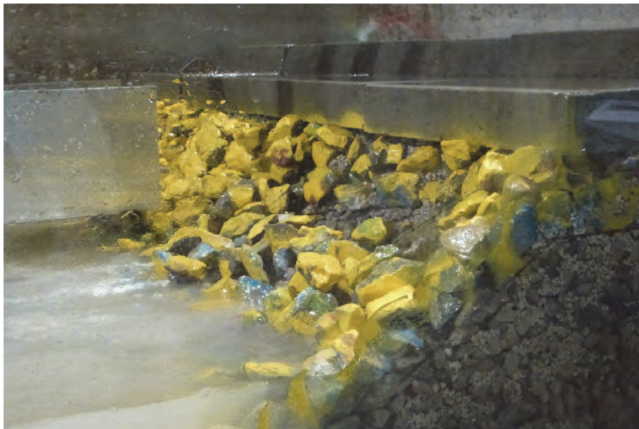
Figure 3.9: Damage to the 0.5-2 t rear side rock of a breakwater by wave overtopping.
