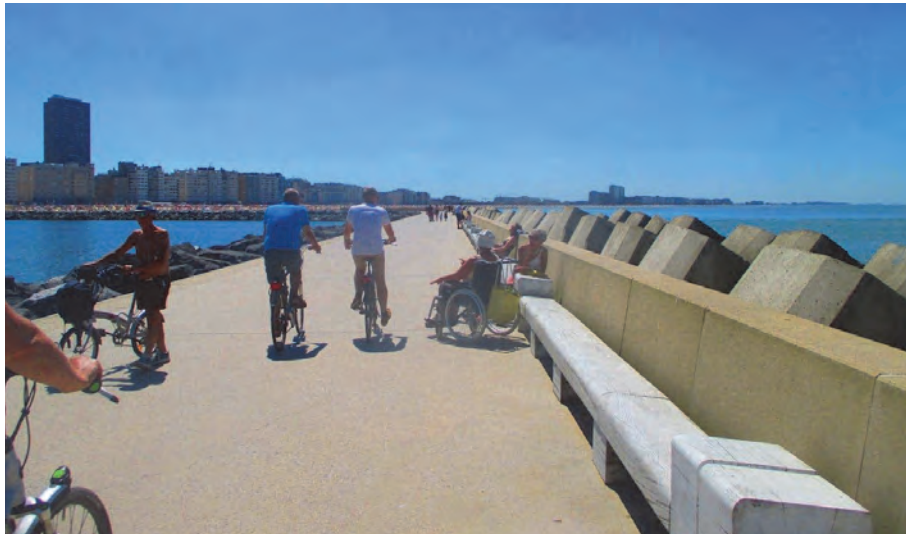
Figure 3.16 New breakwater at Oostende, Belgium, with a main function of access for people
