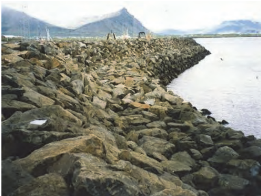
Figure 6.10 Icelandic-type berm breakwater
