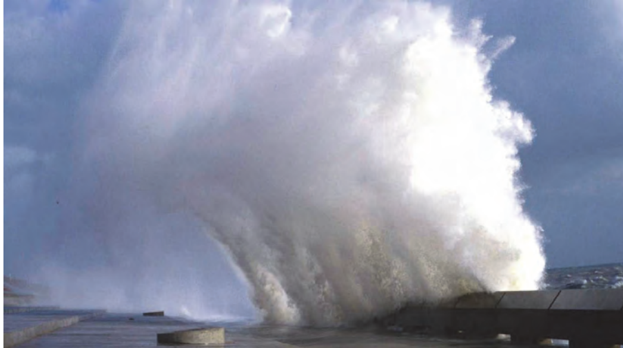
Figure 3.17 Severe wave overtopping at Samphire Hoe, UK.
