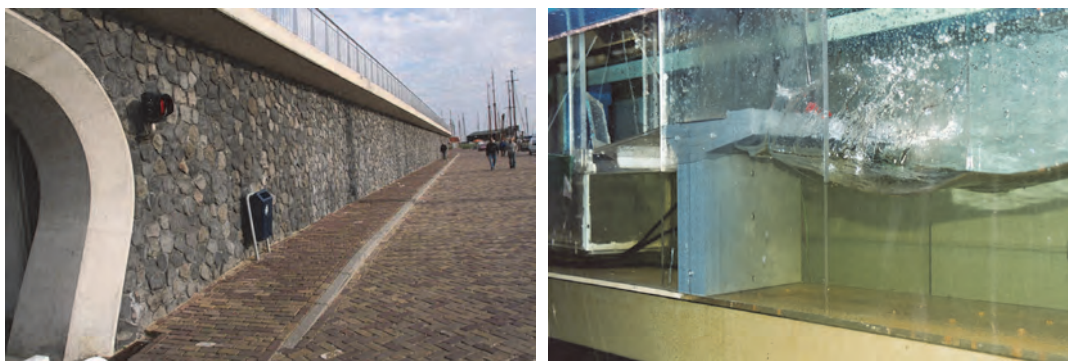
Figure 1.9: Large and effective wave return wall at Harlingen (NL). The wave return wall is part of a promenade on top of the wall (picture above). Lower left: the wall with wave return wall in reality; lower right: model testing under design wave conditions
