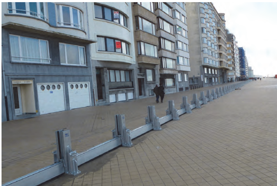
Figure 3.13: Apartments on the boulevard at Oostende, Belgium, protected by a movable storm wall to reduce impacts by overtopping waves
