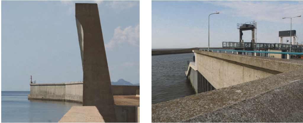
Figure 7.19: An example of a modern, large vertical breakwater with bull nose (left – Carthagena, Spain) and view on a harbour wall with bullnose under daily conditions (right – Harlingen, NL)
