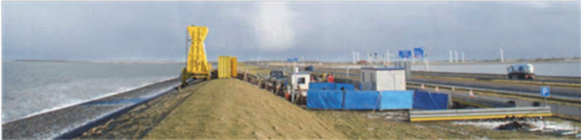
Figure 4.33 Set-up of the Wave Overtopping Simulator close to a highway
