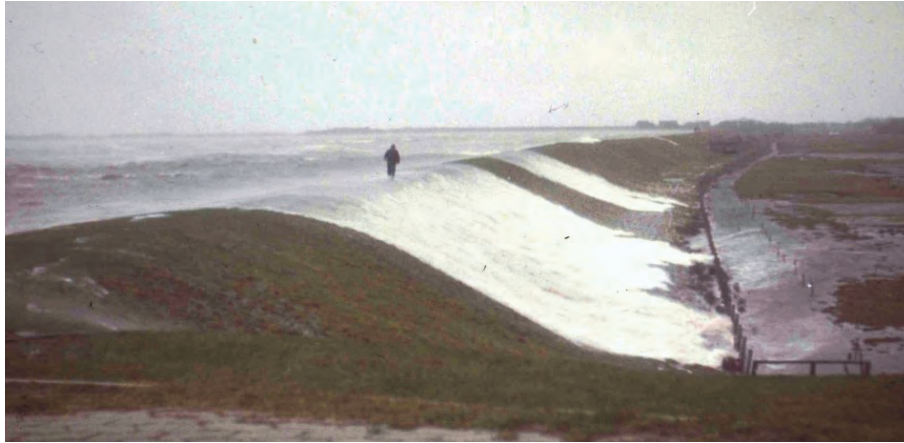
Figure 3.19 Wave overtopping over a sea dike (photo Zitscher)
