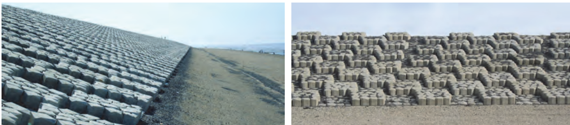
Figure 5.31: Chessboard pattern produced with two thicknesses of placed block revetments. The roughness has only been placed in the run-up zone, above the wide asphalt berm
