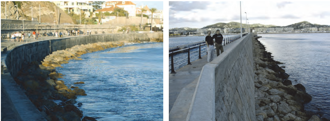
Figure 7.13: Examples of composite vertical structures, Barcelona, Spain (left), Ibiza (Spain) right
