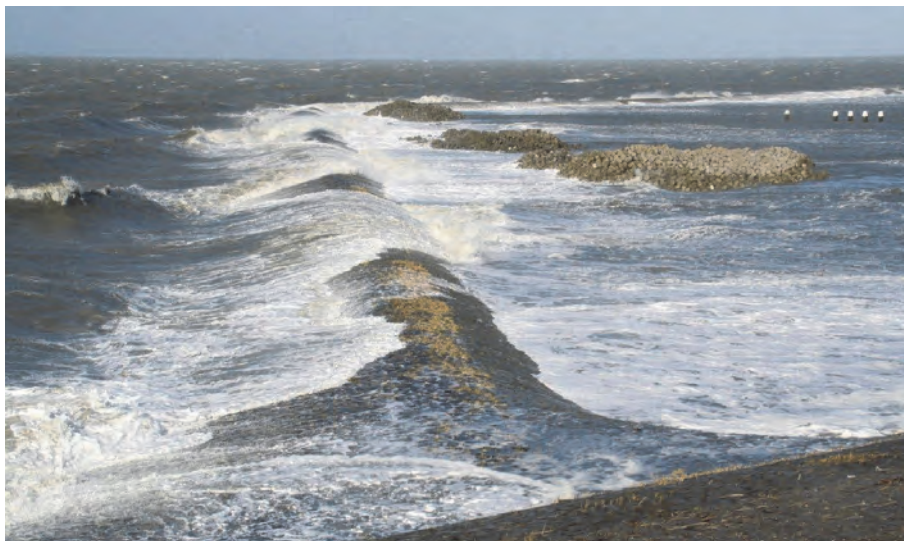
Figure 3.20 Dangerous overtopping over a smooth low-crested structure. Near locks at Afsluitdijk, NL
