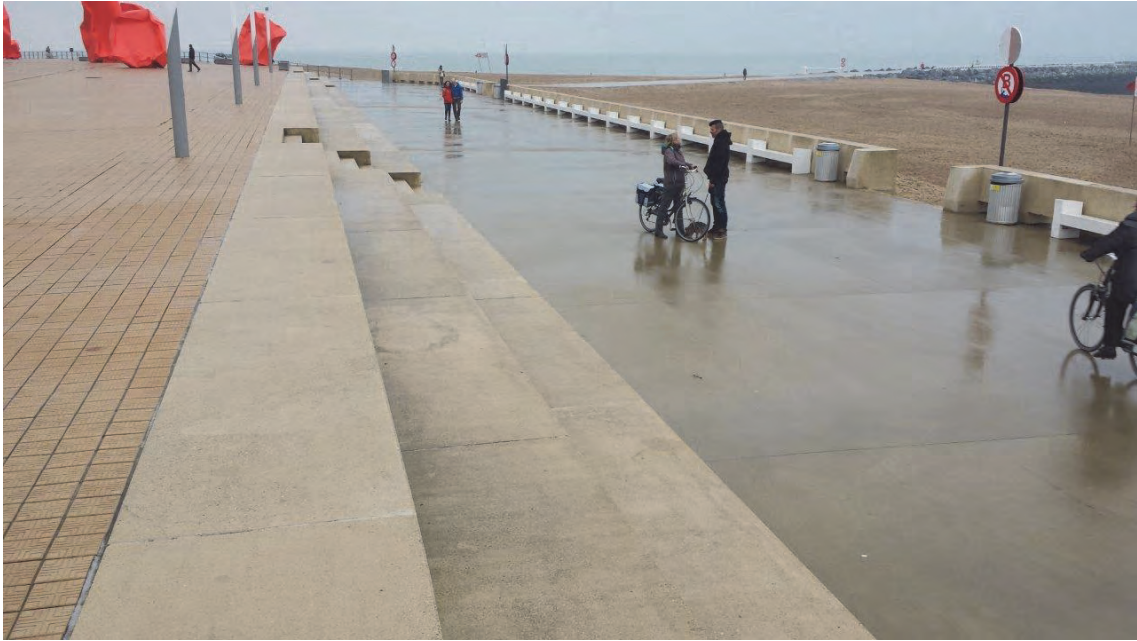
Figure 5.52: A stilling wave basin at Oostende, BE
