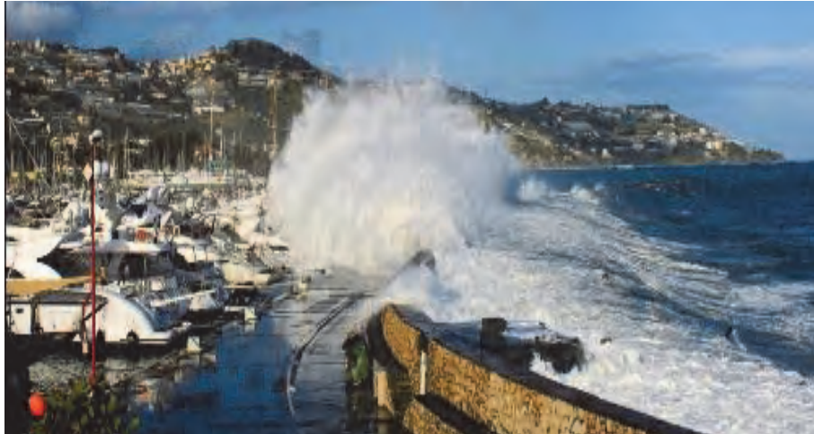
Figure 3.12: Wave overtopping at the marina of San Remo, Italy, damaging small boats
