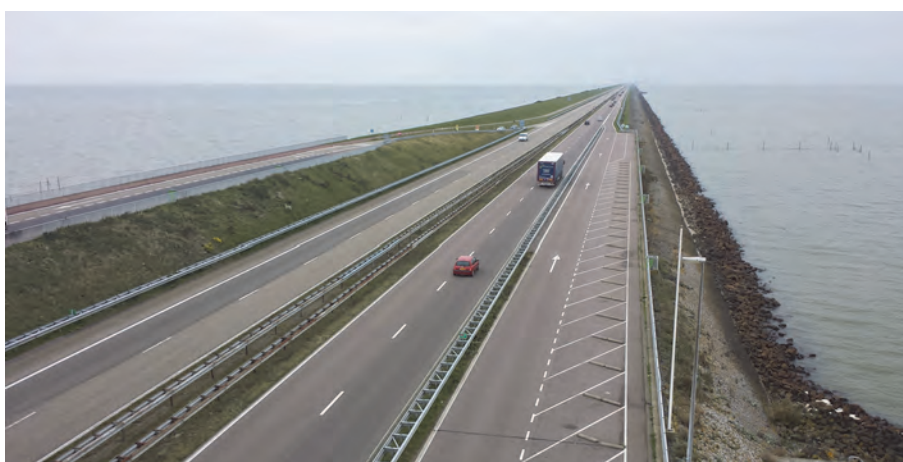
Figure 3.22: The highway on the Afsluitdijk, the Netherlands, with the Wadden Sea and the sea defence on the left side and the fresh water lake, the IJsselmeer, on the right side
