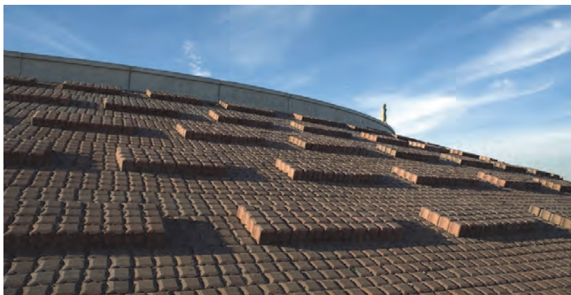
Figure 5.32: Rib pattern produced with two thicknesses of place block revetments. Each area of 4 by 5 units is placed mechanically in one move. Courtesy Projectbureau Zeeweringen
