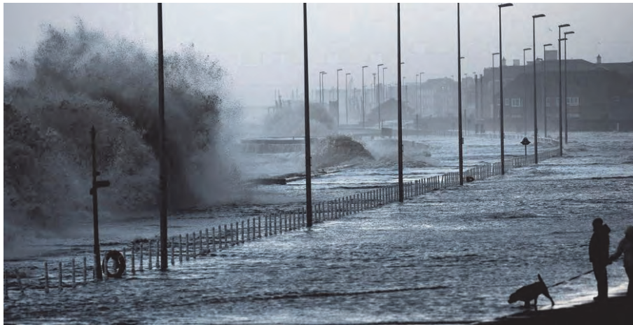
Figure 3.21 Wave overtopping at a seawall with a wide boulevard
