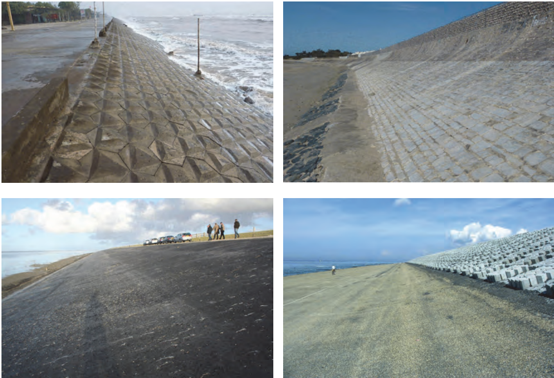
Figure 5.2: Examples of coastal dikes, levees and seawalls. Hanoi, Vietnam; Ile de Ré, FR; Boonweg, NL; Hondsbossche zeevering, NL
