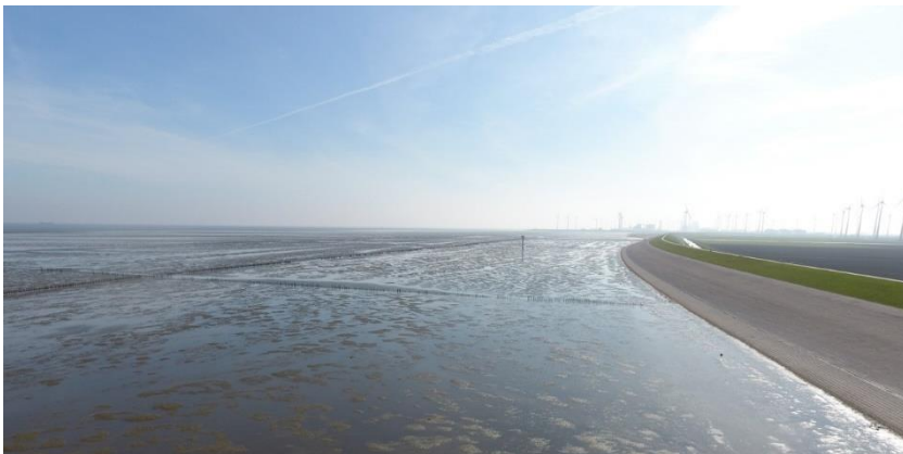
Figure 1.1: Dike partially covered by asphalt and partially by grass, fronted by a shallow, mildly-sloping foreshore (mudflat) along the Dutch Wadden Sea coast.
