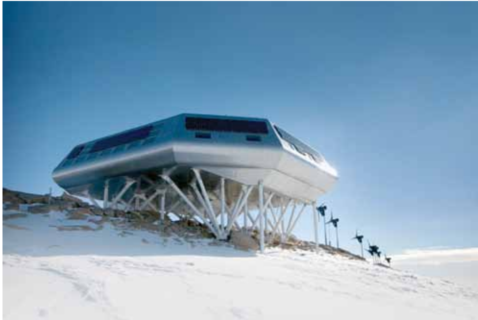
Fig. 5.1-3 Antarctic Station Princess Elisabeth, Belgium, located at 71°57' S 23°20' E.
