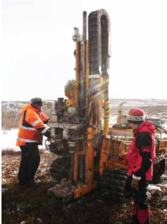
Fig. 2.9-2. A small moving drill was used to make holes to measure permafrost temperature for the BTF and PYRN-TSP projects near Abisko, northern Sweden. (Photo: Frida Keuper)
