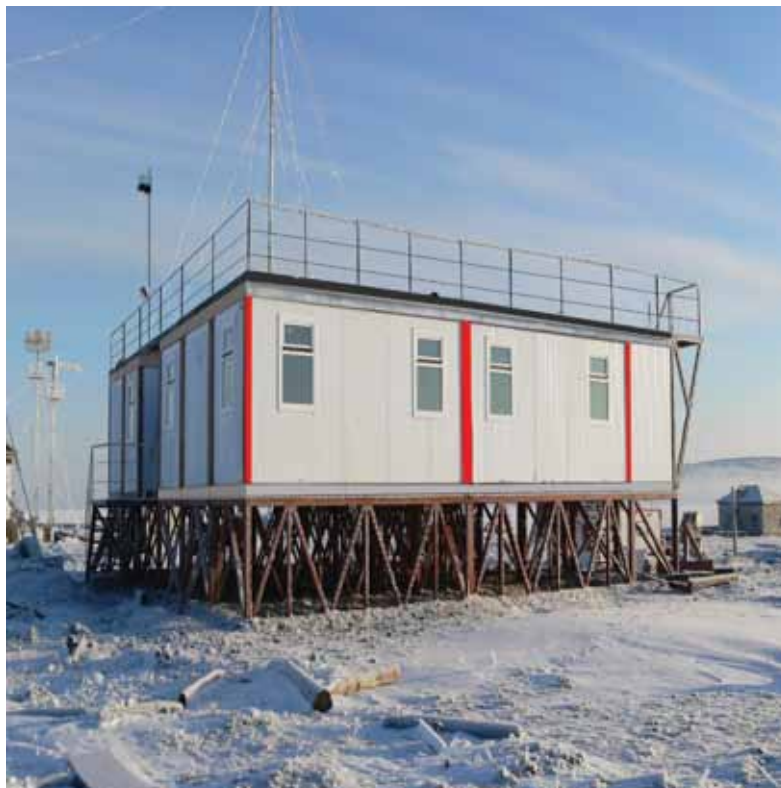
Fig. 2.1-1. The new building of Tiksi Observatory.
