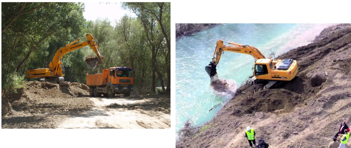
Fig. A2.2.2. (a) Removal of embankments to reconnect riverbed and floodplains in Natura2000 sites; (b) embankment removal and reintroduction of sediments - in some cases, performed by the same operators which decades ago had dredged the river and constructed the berms (Source: Gov. Navarre & MN Consultors).
