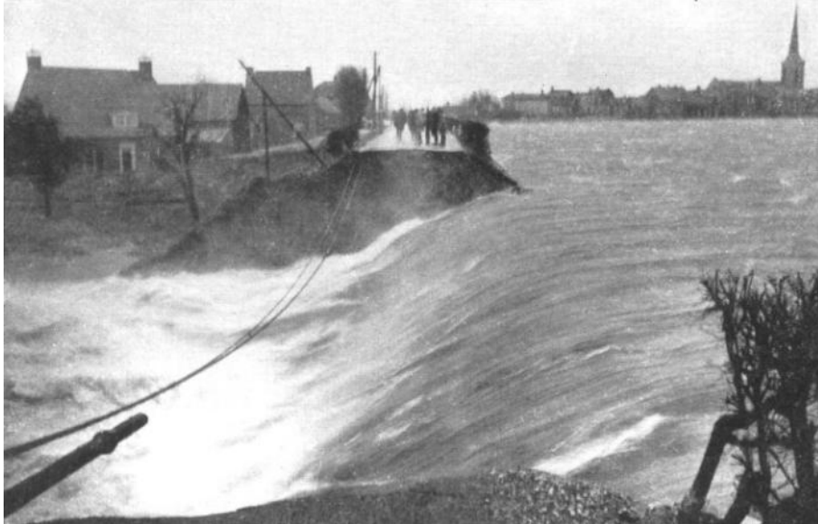
Figure 1.2 A levee breach (Ouderkerk aan de IJssel) during North Sea storm surge of 1953 (source: Van Veen 1962)
