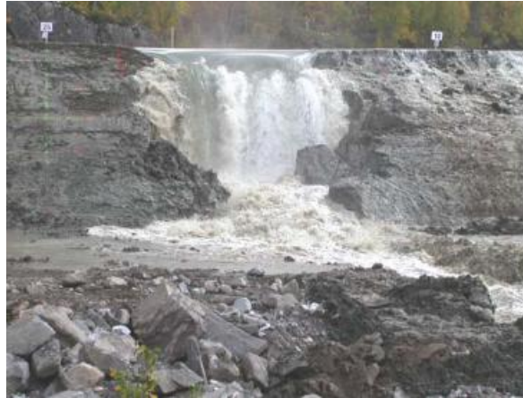
Figure 1.9 Breach formation in a cohesive embankment (IMPACT Project, form Morris & Hassan (2009))
