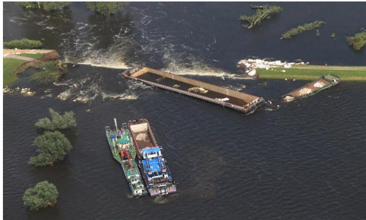
Figure 1.4 Deliberate sinking of three barges to close a breach in the Elbe River levee during the 2013 floods. This reactive measure was used to obstruct the torrent and allow for permanent repairs to the failed dike system near Fischbeck (source: www.spiegel.de ).
