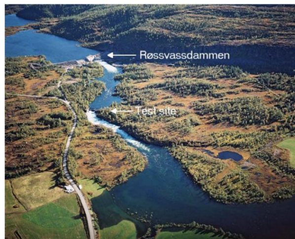
Figure 1.12 Aerial view of the Røssvass dam breach test site of IMPACT project (Source: Løvoll et al (2004))
