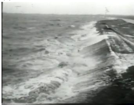
Figure 1.7 Hydraulic loads including: (a) river overflowing (river-side view) (b) wave runup (sea-side view) and (c) wave overtopping (land-side view)
