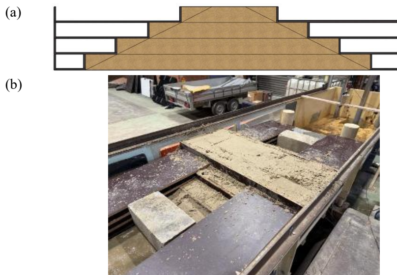
Figure 6.7 Custom lateral support system and embankment construction: (a) schematic design and (b) embankment configuration in practice prior to final slope shaping.
