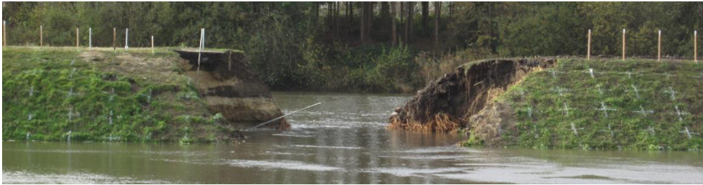
Figure 5-6 Breach 18/11/2015
