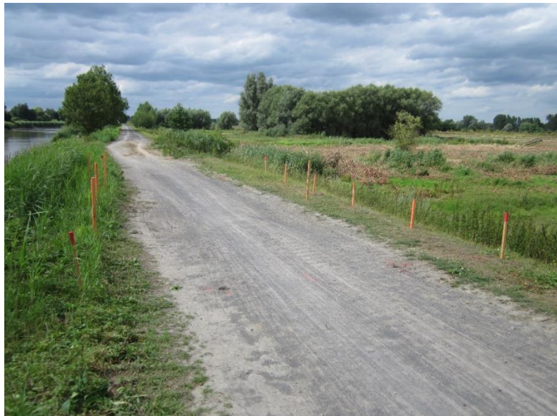
Figure 1-5 Dike at location breach experiment
