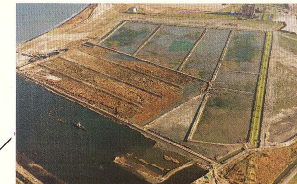
Natural processes for the fast dewatering of dredged silt
