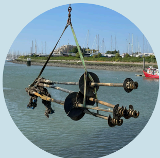
5 out of 6 backbones were anchored by means of large screw anchors.
