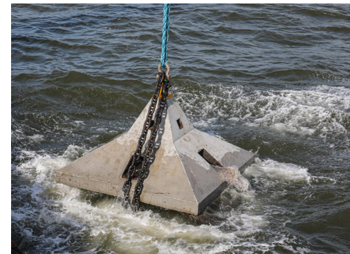
Bio-facilitating anchor during installation.
