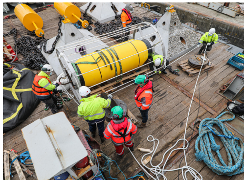
Mussel shaker and bio-facilitating anchors on deck of the installation vessel.
