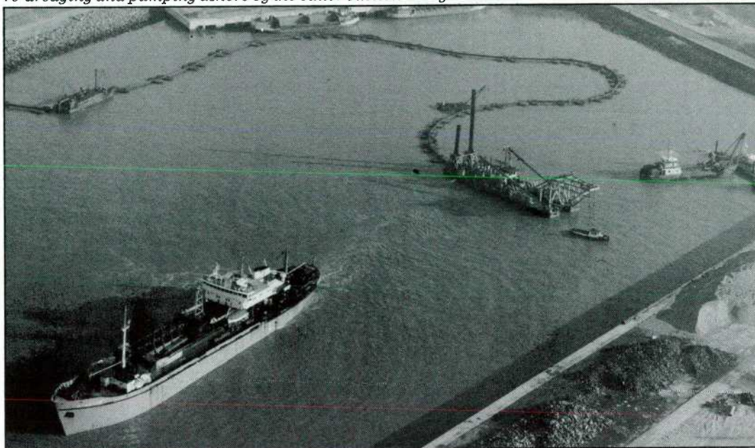
The trailing-suction hopper dredger "Atlantique" is pictured here dumping its sand load for re-dredging and pumping ashore by the cutter suction dredger "Brabo".
