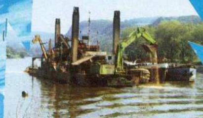
Rock and gravel dredging
