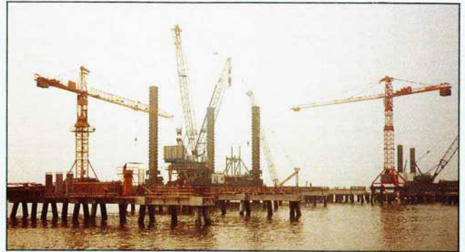
Begemac N.V. of Antwerp supplied longitudinally welded steel pilings with an outside diameter of 914.3 × 14 mm wall thickness and in different lengths of between 25,050 and 28,790 mm for the LNG terminal (as shown in the photo). The company also supplied longitudinally welded tubular steel dolphins with a diameter of 2,200 mm and in different wall thicknesses of between 25 and 58 mm.
