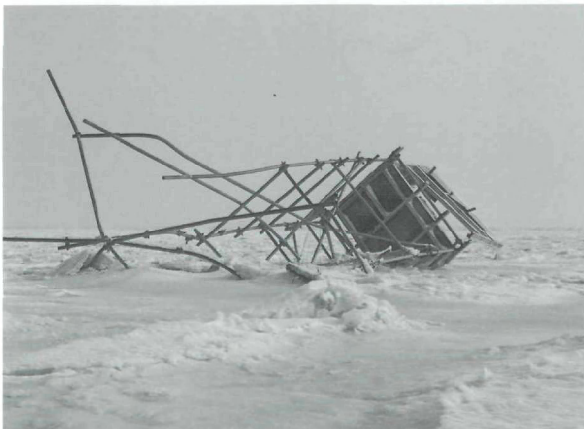
The observation towers on the tidal flats were strong enough to resist winds with hurricane force and storm tides, but the force of drifting ice was too much. Hence we had to rebuild the towers after every severe winter.
