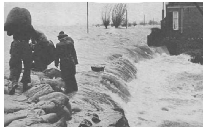
fig. 23 Breached dyke in February 1953
