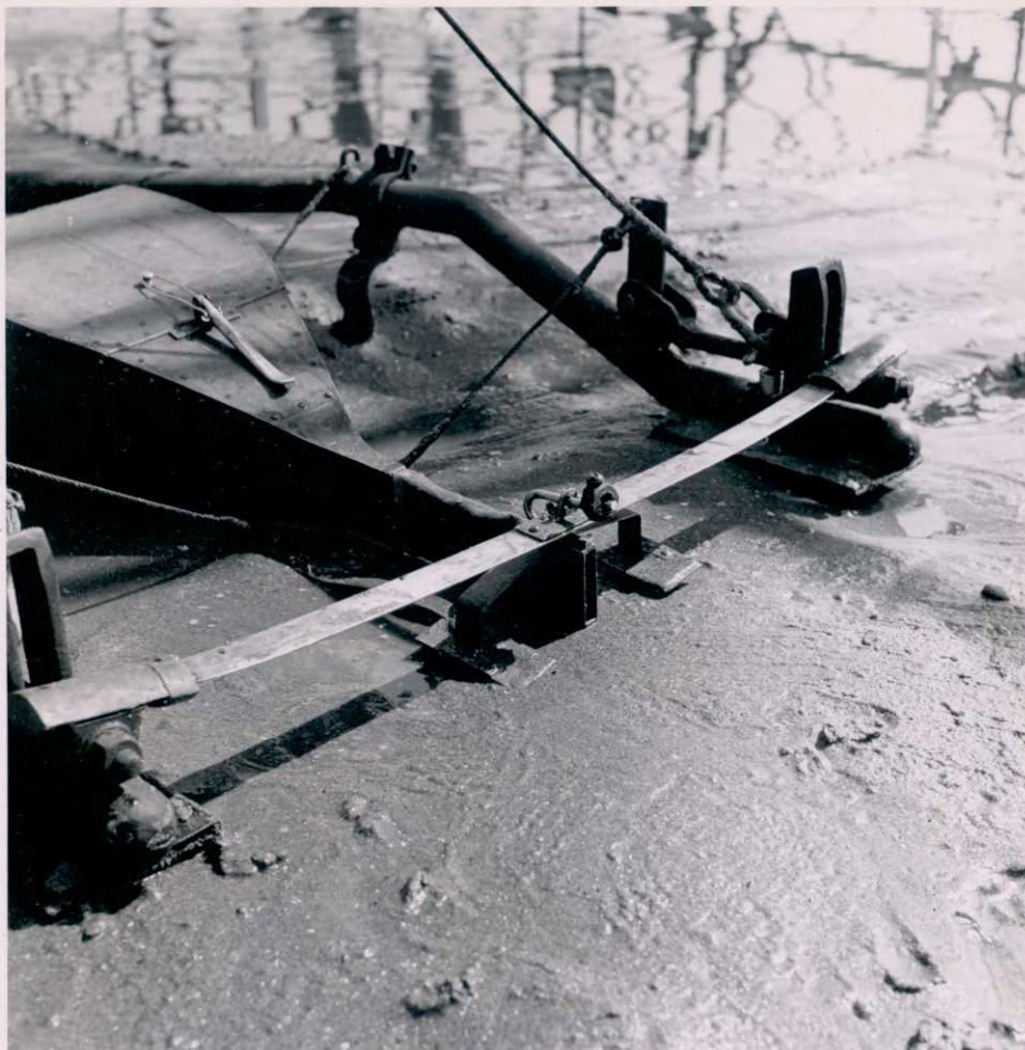
5. BODEMTRANSPORTMETER „SPHINX“ DETAIL INSTROOMOPENING (55.f.84)
