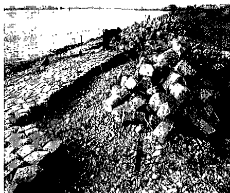
Outer berm of a dike protected by polygone concrete blocks
