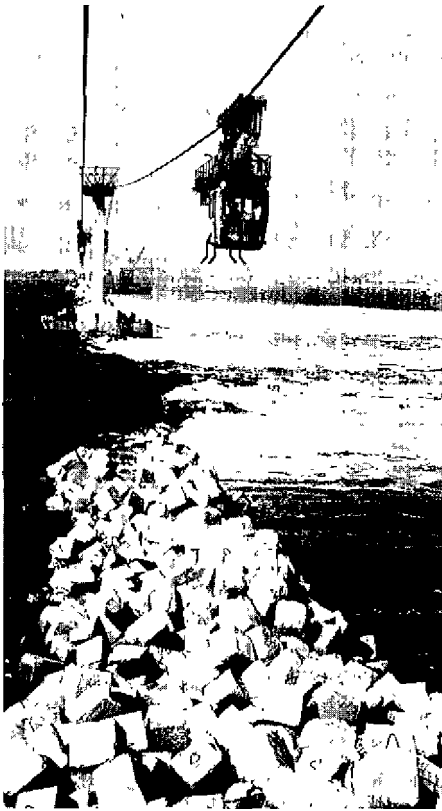
Cable railway for dike construction
