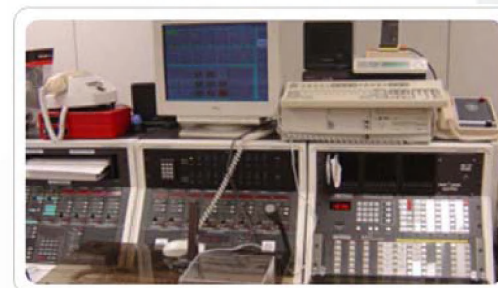
Command module for emergency siren alert broadcasting system, Oahu County Civil Defense Agency, Hawaii. Credit: ITIC
