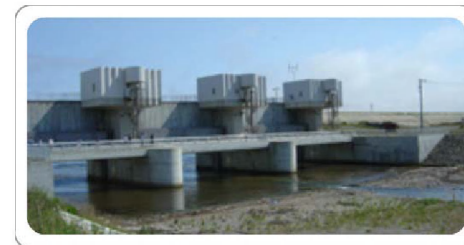
Water gate used to protect against tsunami waves on Okushiri Island, Japan. The gate begins to automatically close within seconds after earthquake shaking triggers its seismic sensors. Photo courtesy of ITIC.
