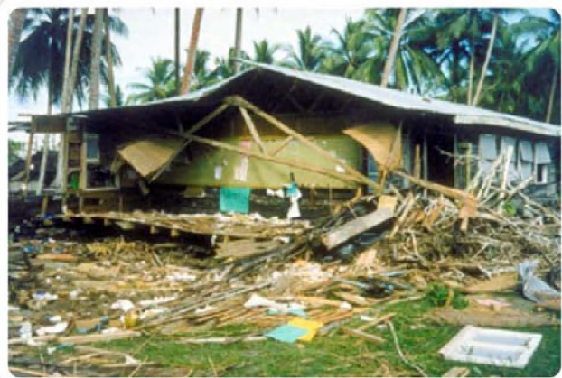
A two-story wooden school building that stood near the church at Sissano Mission was carried 65 m by the wave until caught by a grove of coconut palms. The lower floor of the building collapsed, but the upper floor class rooms were preserved. Schoolwork was still hanging on the wall. (Photo credit: Hugh Davies, University of PNG.)
