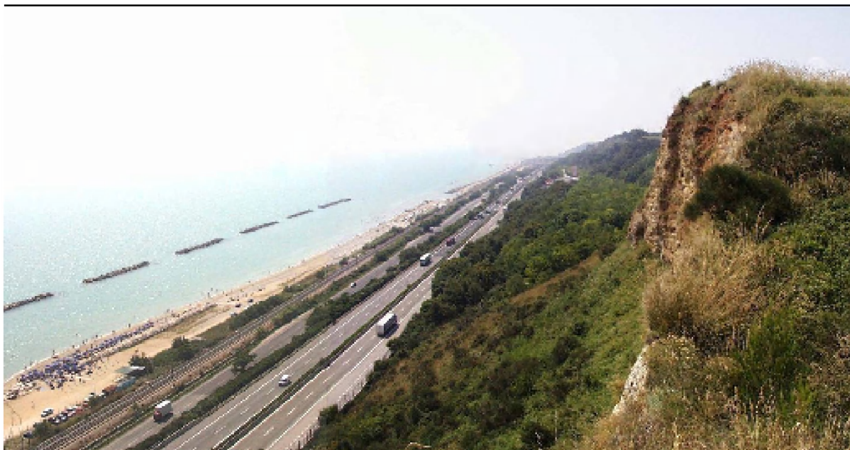
Coastal infrastructure, coastal defences and rockfall risk at Pedaso, Regione Marche, Italy
