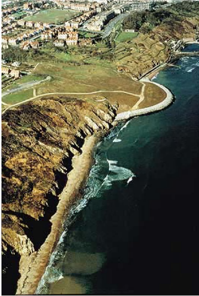
Holbeck Hall landslide after remediation works were completed, North Yorkshire, UK.
