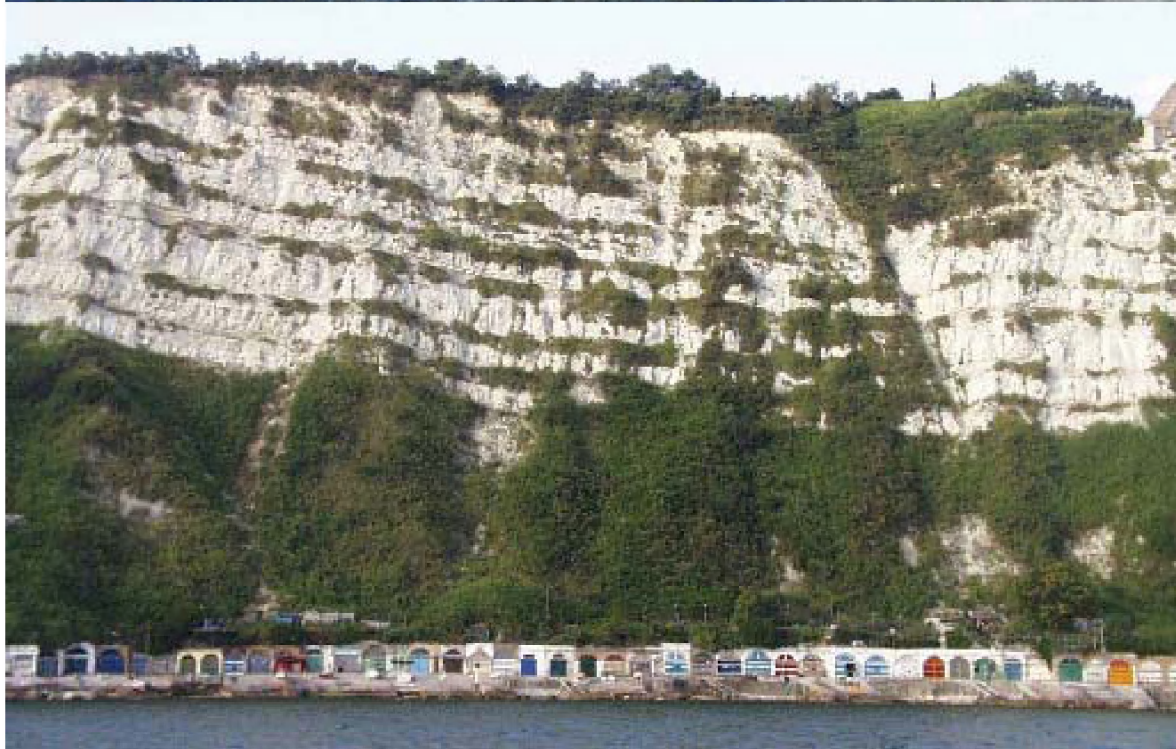
Cliffs of Regione Marche, Italy, with rockfall risk to cliff foot development and industry.
