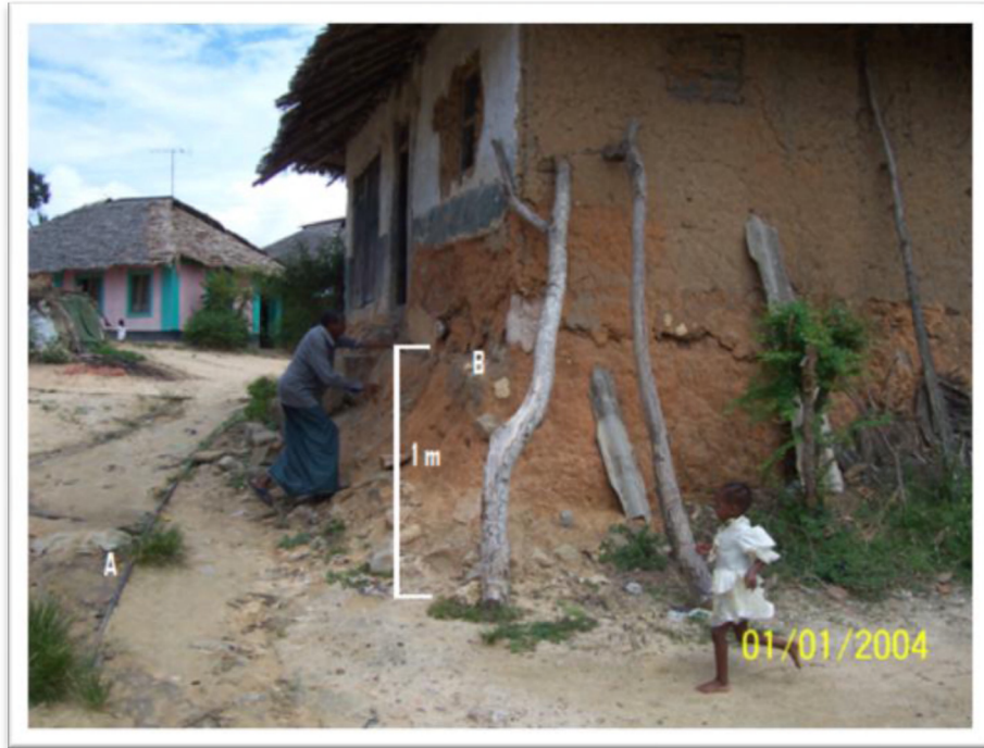
Figure 7.4: Signs of erosion in Jomvu village. The point marked B (Notice the man pointing) is claimed to be the ground level 50-60 years ago when the house was being built. The point marked A is a water pipe that is usually buried more than 1m below the surface. This pipe was installed in the 1960's (Photo taken during study in 2004).
