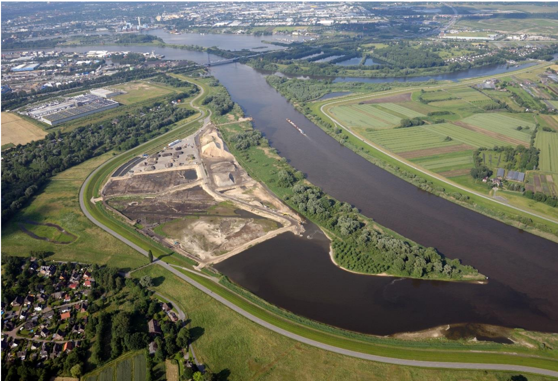
Fig 2: Present status of construction works
