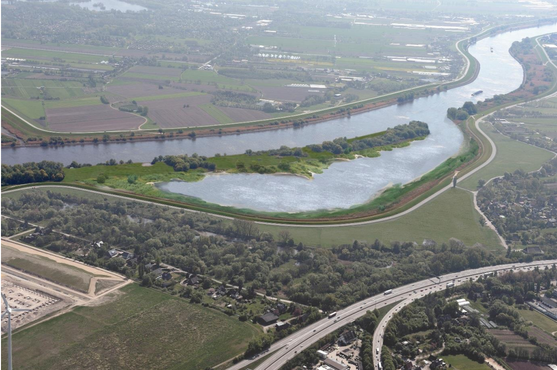
Fig 1: Vision of Kreditsand new shallow water area after completion
