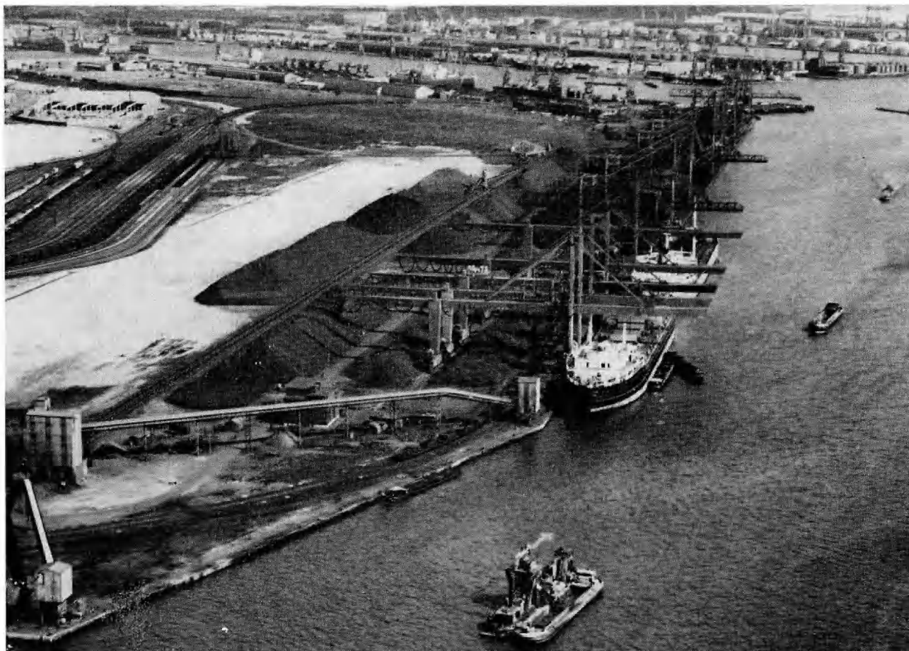
Aerial photograph of the quay in operation
